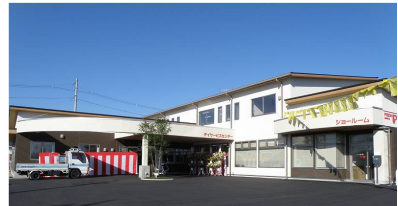
Relocation of Pigeon Manaka main headquarters and launch of day services
